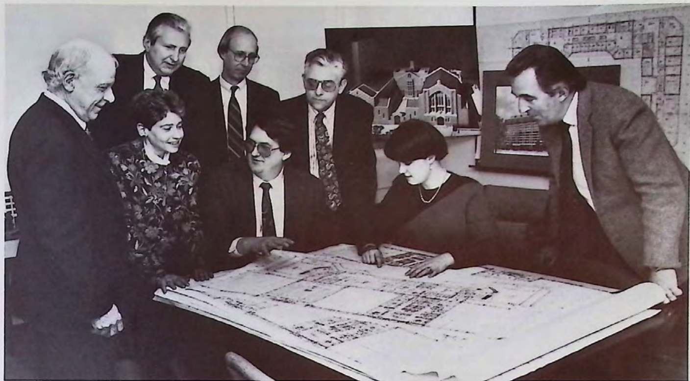
After the District of Columbia's Zoning Commission and Historic Preservation Review Board approved, respectively, the Fund's zoning request and denied a neighborhood's group's petition to grant historic landmark status to the Western Presbyterian Church, the way was cleared for construction to begin on the new church. Involved in the project are (from left to right) Al Harper, Chief of the International Square Facility Unit; Joan Powers, the Fund's administrative lawyer; Bruce Hobbs, Chief of the Administrative Services Division; Peter Gerridge, Senior Service Officer of the Project Support Unit; Geoffrey Vaughan, Deputy Division Chief of the Administrative Services Division; Jim Kalser, Advisor in the Administration Department; Sue Hern, Deputy Chief of the International Square Facility Unit; and Tim Cole, Assistant Director of the Administration Department.
