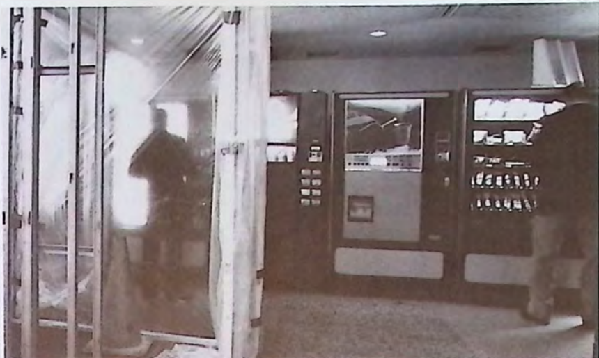
The vending machines will remain in operation throughout the renovation of the vending area on the Concourse Level.
