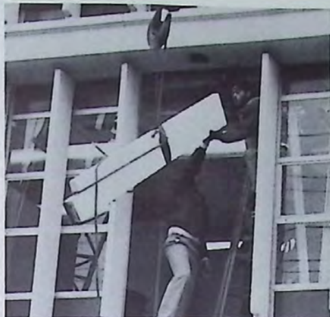
With the slab dislodged (above), a crane is used to transport the IBM equipment to a waiting moving van (right).
