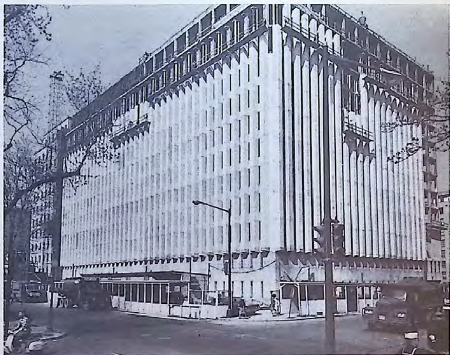
"The Addition" is shown here as photographed at an advanced stage of construction earlier this month. The view is from 19th and G Sts. facing north-east.
